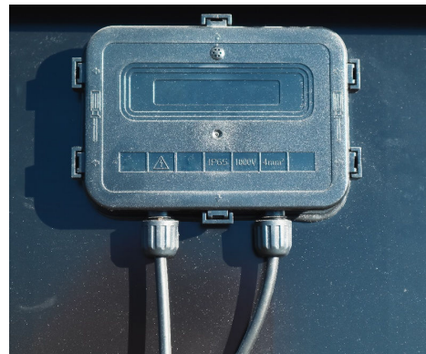
(b) junction box behind module
